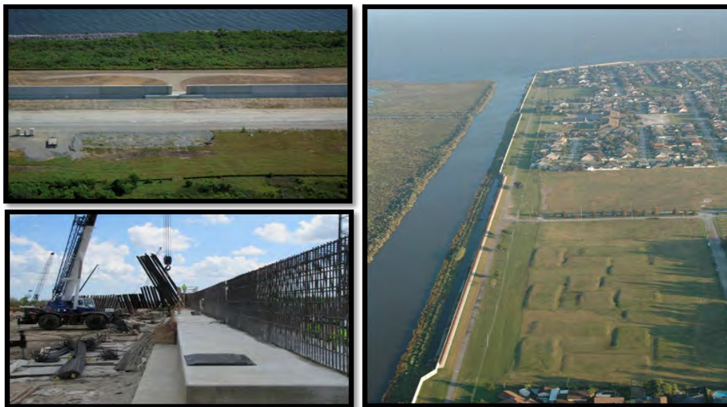
Photograph 4-1. Examples of floodwalls and levees with floodwall caps.
