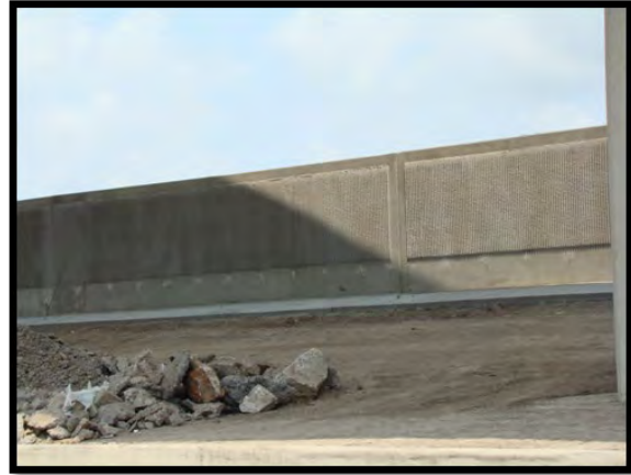
Photograph 4-3. Aesthetic articulated fin finish for floodwalls at the Franklin Ramp.
