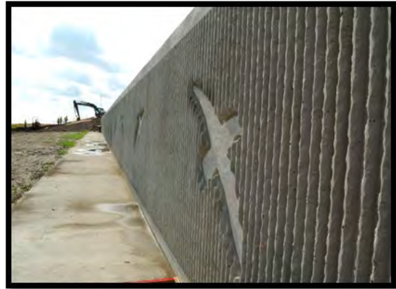
Photograph 4-2. Aesthetic concrete stamping for floodwalls at the Williams Boat Launch.
